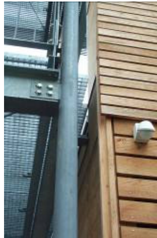
Figure 2.7: Spaced and ventilated timber cladding
